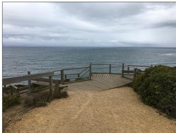
Above: Upgrading at the Southside Visitor area at Pt Addis includes the boardwalk and all abilities access to the lookout.
